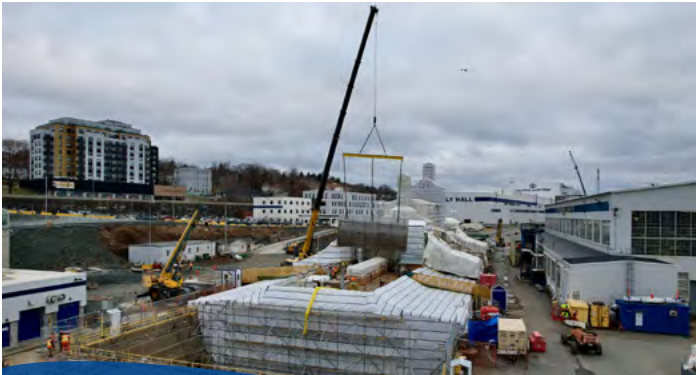
Aft Engine Room Insert for HMCS Halifax
